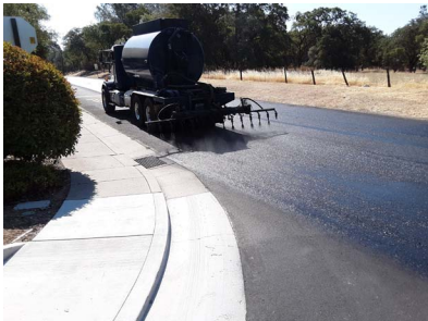
Spray application of TRMSS – without the common brown-to-black color change. The distributor
