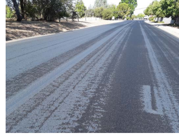
TRMSS cure stages (L at 20 min; C at 10 min; R at 5 min.)
