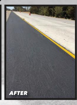
**THE EDGE SEAL** system replaces old technology and the slow, labor-intensive methods of fixing, filling and sealing damage along the joint edge.
